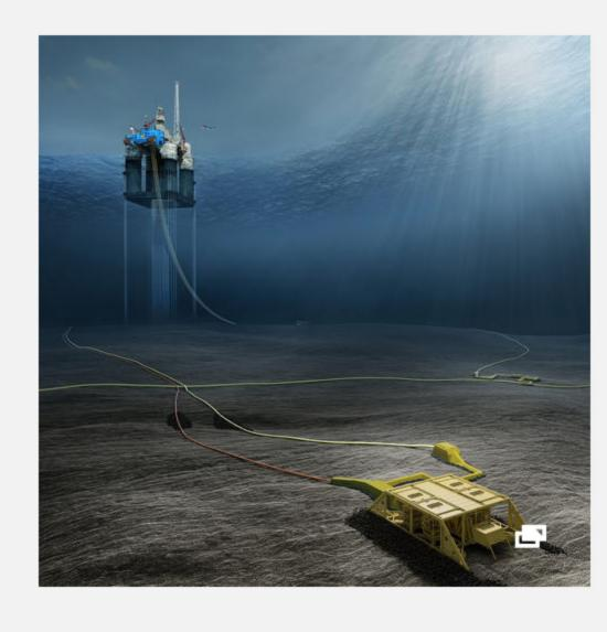
Dvalin will be developed with a four wells subsea template, which is connected to the Heidrun platform. At Heidrun, the gas will be partly processed in a new module, before the gas is transported in a new export pipeline to Polarled, going to the Nyhamna onshore gas terminal. At Nyhamna, the gas will be processed and transported to the European market.
