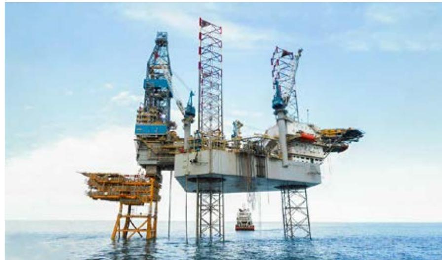
◀ Vega Pléyade is connected to the onshore processing installations at Rio Cullen via a 77-kilometre gas exporting pipeline.
