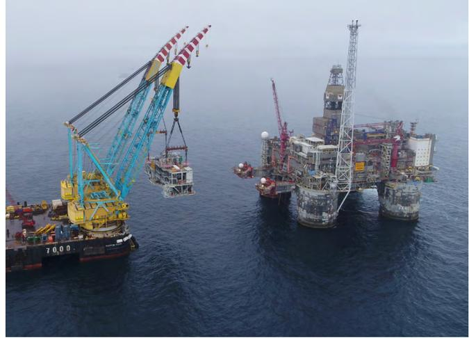
The heavy lifting vessel Saipem lifts the Dvalin module onto the Heidrun platform.
